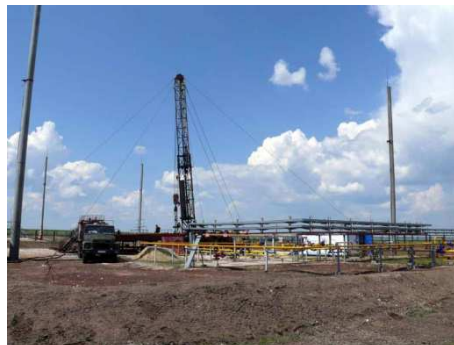
VM#1 well workover in operation
